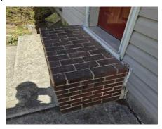
• Porch Settlement Observed. The soil below the porch has settled. Minor settlement may occur over the life of a porch and is not considered a structural defect. Resurfacing, leveling or patching may be necessary to correct the deficiency. If significant, it is suggested to have a qualified specialist further evaluate and make corrections as needed.
