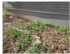
• Vegetation In Contact With The Structure. All vegetations should be trimmed away from the structure. It is suggested to have a qualified specialist make corrections as needed.
