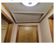
• Attic ceiling hatch trim is loose, suggest corrections to secure.
