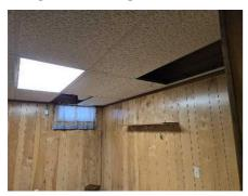
• Some suspended ceiling tiles missing or damaged, suggest corrections
