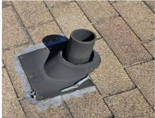
• Roof Pipe Flashing Rusted. Pipe flashing, sometimes referred to as a roof boot, is manufactured to seal tightly around small ventilation pipes, plumbing, and other vents and equipment that protrude from the roof of a home or commercial building. The flashing is necessary to prevent leaks. The base is typically a flexible metal so that it is compatible with virtually any roofing material. It is suggested monitor the roof pipe flashing in the future and make corrections as needed.
