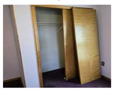
· Closet bypass doors need adjustments throughout, off track, dragging on floor, missing floor guides.
