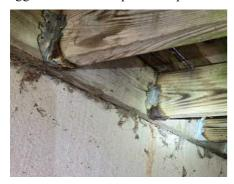
• Improper Joist Hanger Fasteners Installed. Current fasteners are not intended for use in hangers. Every hole in a structural hanger should be filled with an approved structural fastener/ screw or nail. It is suggested to have a qualified specialist make corrections as needed.
