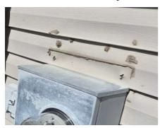
• Seal holes in siding above current meter, likely from previous meter location.
