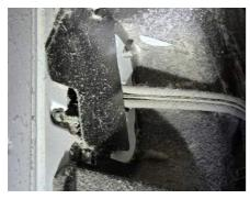
• Missing clamp on chord at back of dryer, suggest install to protect from vibration.
