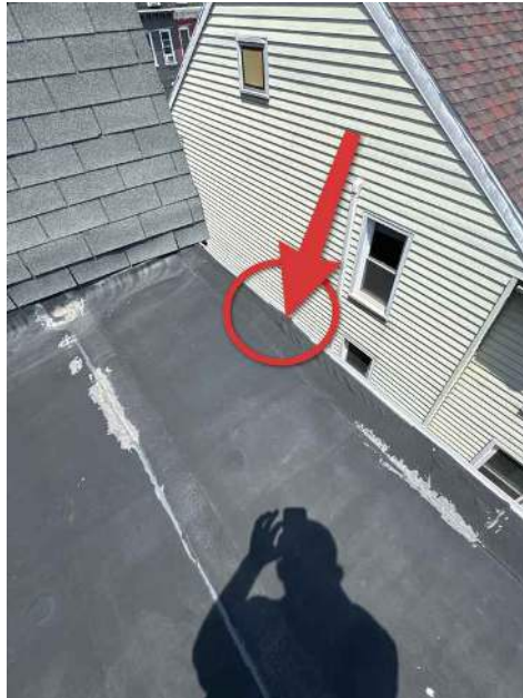
Hole in rubber edge seam
