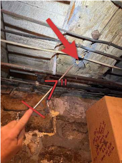
Screwdriver plunged all the way through beam
