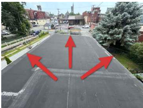
No railings around roof edge
