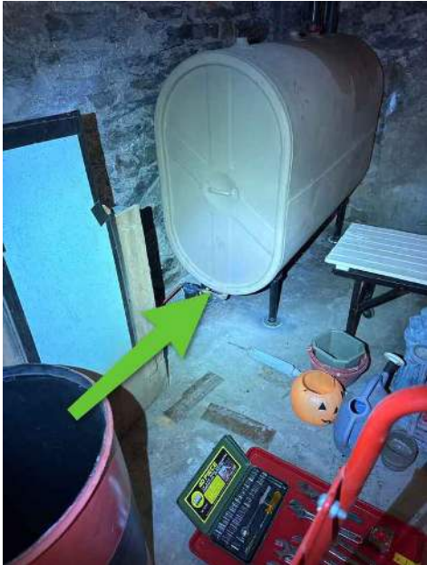
Oil shut off valve
