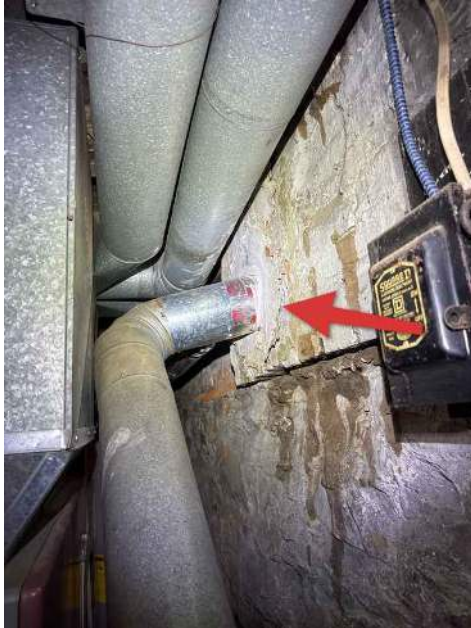
Seal around vent delaminating
