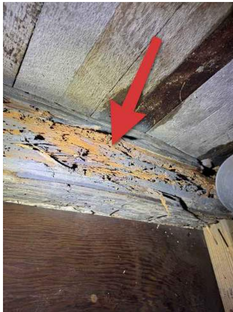
Wood damaged by termites
