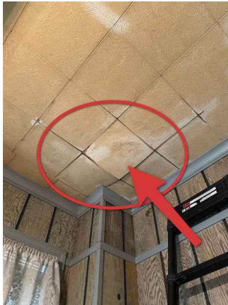
Ceiling damaged by moisture
