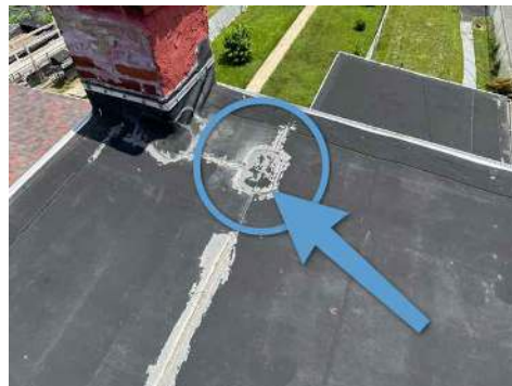
Caulk needed around patch
