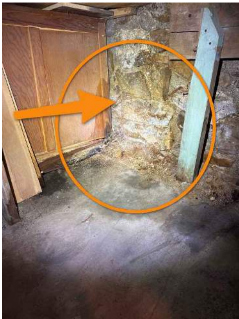
Close up - moisture appears to be seeping through foundation wall
