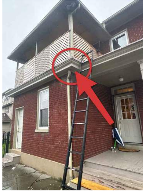
Wood soffit rotted
