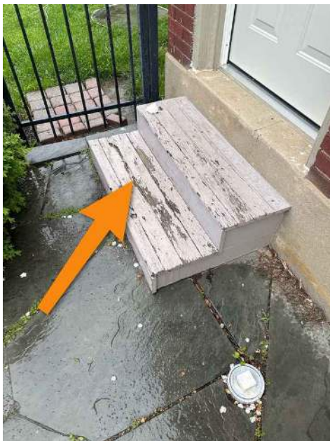
Step boards beginning to rot
