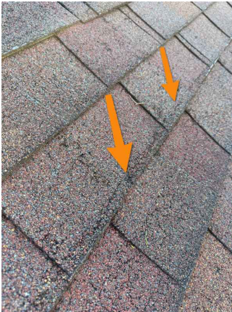
Shingle cracking
