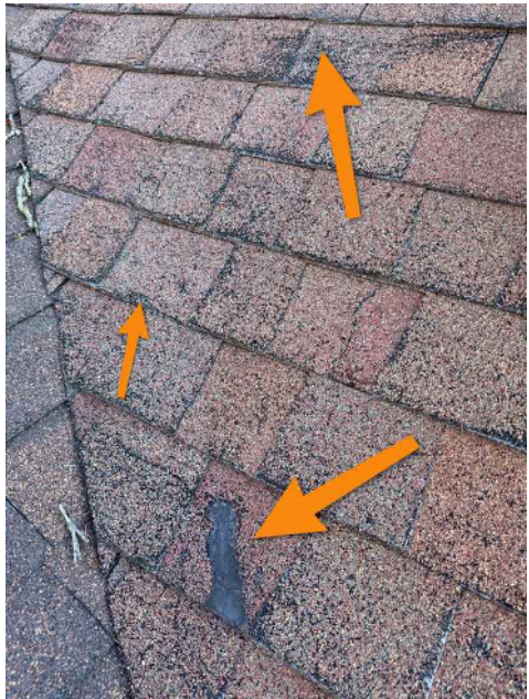
Shingle damage and wear
