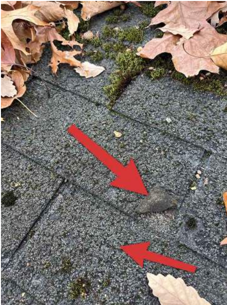
Brittle and cracked shingles
