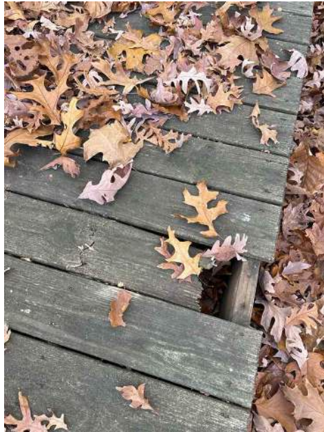
Damaged decking
