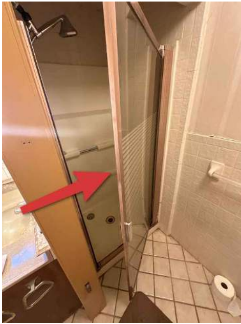
Corroded metal
