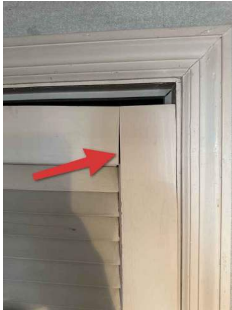
Close up spilt joint
