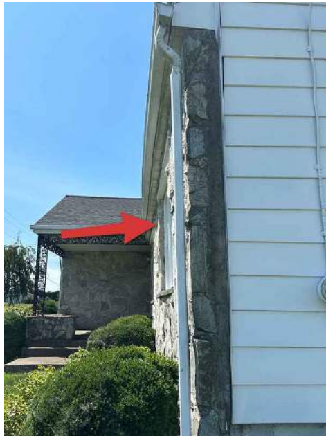
Front Wall Exterior
