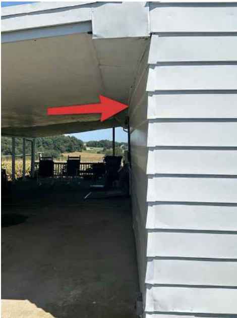
Rear Wall Exterior
