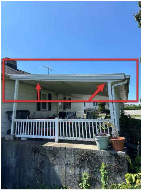
Porch ceiling and support structure
