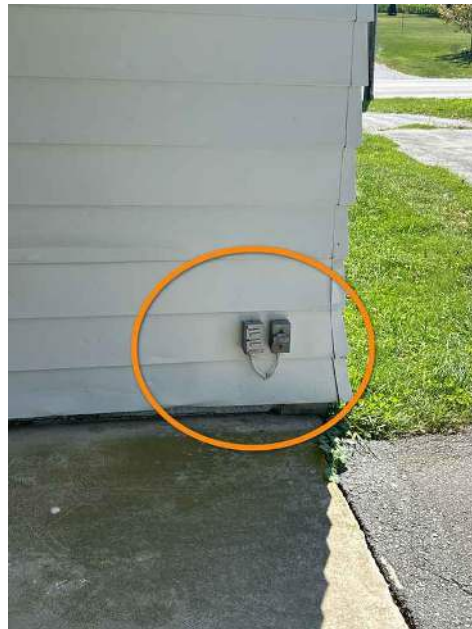
Rear Corner Carport
