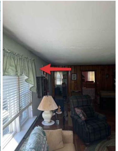
Front Wall Interior
