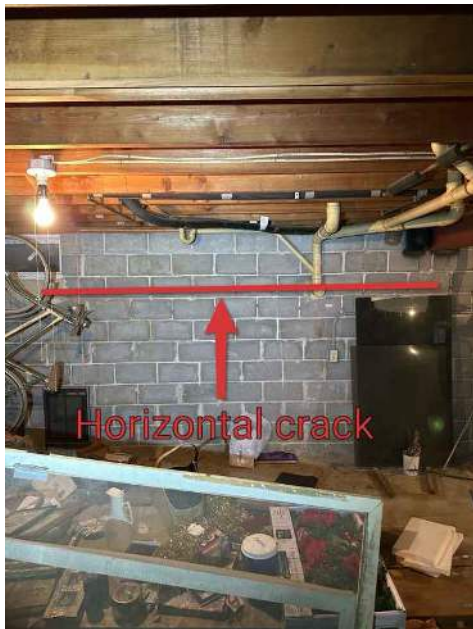
Left Side Foundation Wall Perspective view
