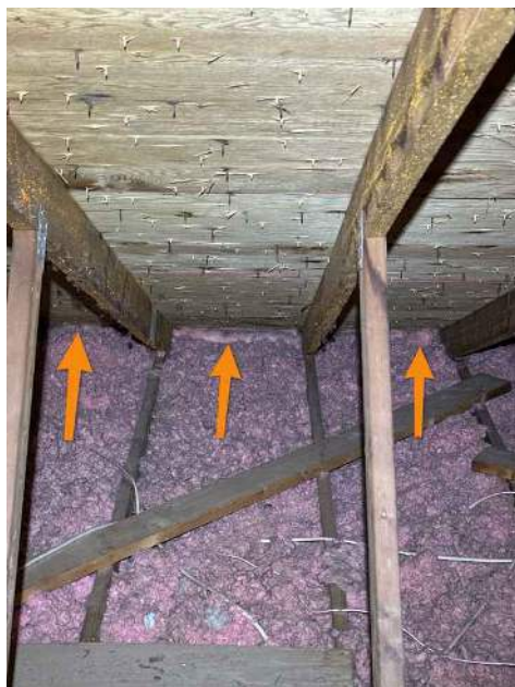
All along rear soffit
