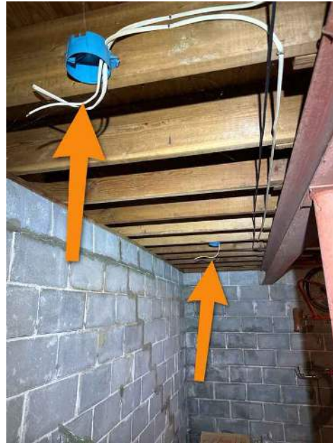
Front Foundation Wall Ceiling
