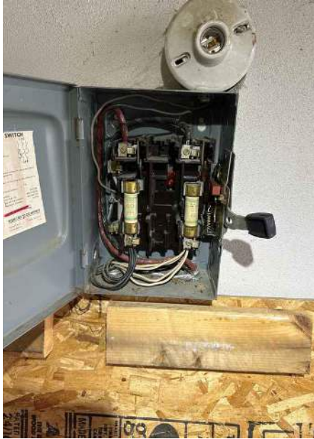
60 amp barrel disconnect AC
