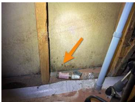
Close-up front basement
