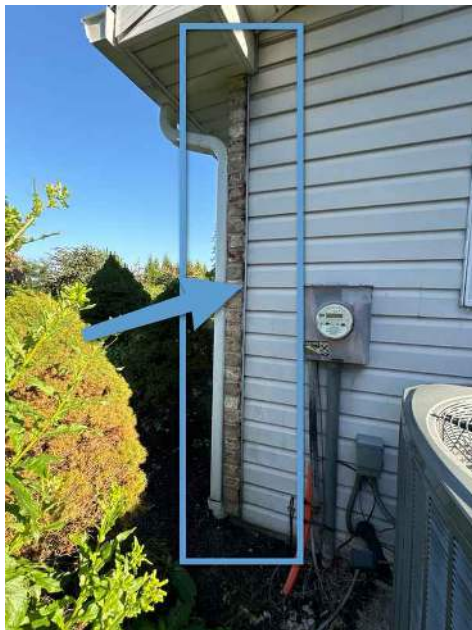
Gap between brick and aluminum siding
