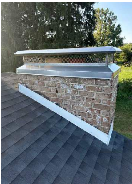
Right Side Chimney
