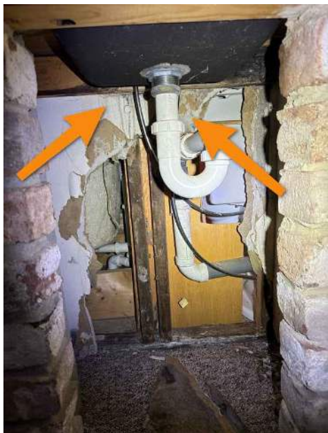
Close up - basement bar
