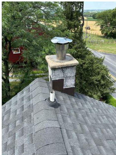
Front Right Side Foyer Chimney
