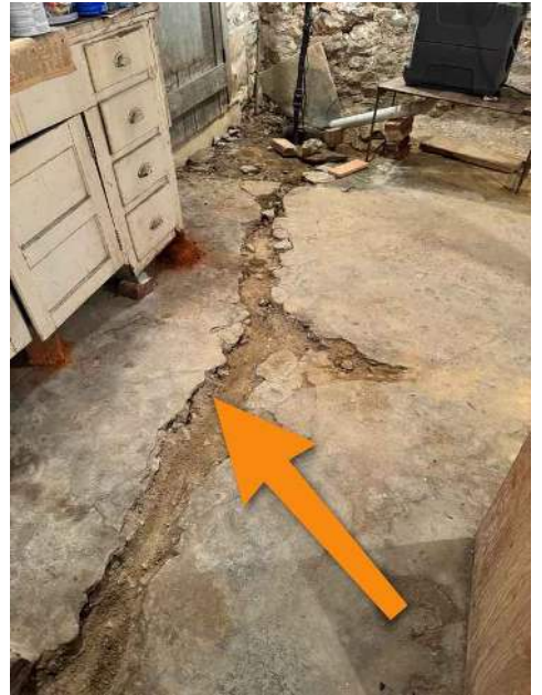
Trenching to direct water to sump pit
