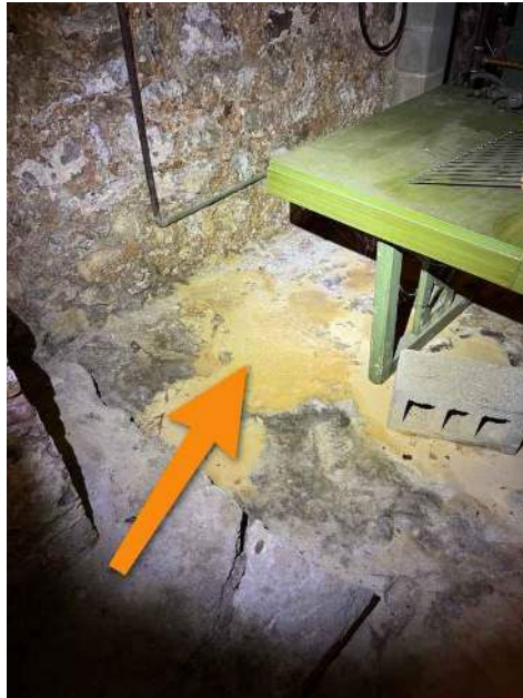
Rear Right Side Basement
