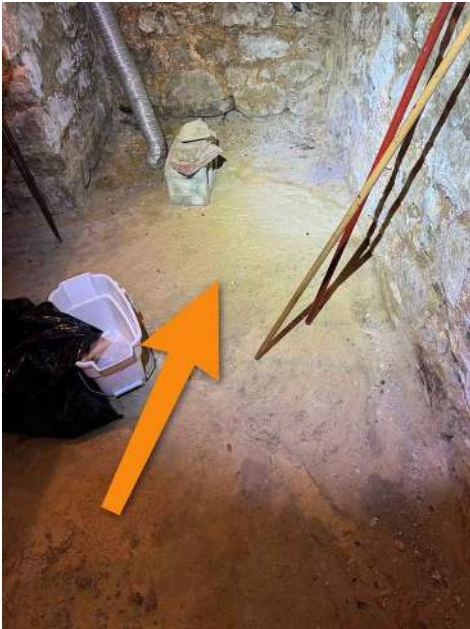
Rear Left Side Basement
