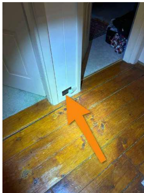
2nd Floor Hall
