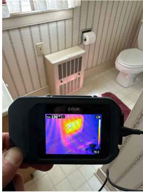
2nd Floor Bathroom
