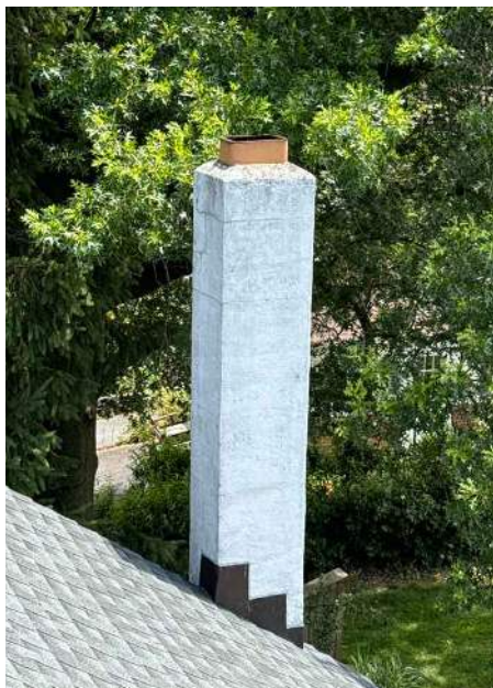
Rear Left Side Chimney
