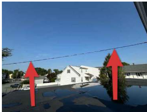
Power cable too close to roof
