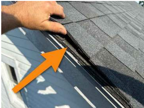
Multiple roof layers
