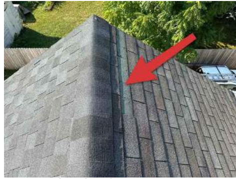
Missing shingle tabs
