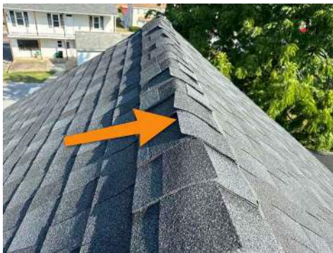
Not designed for Ridge application
