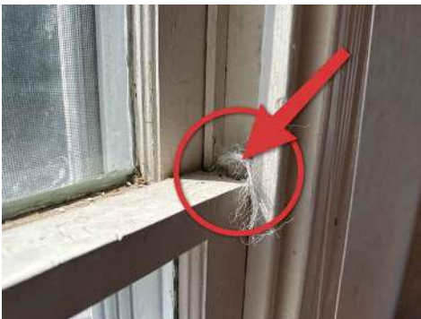
Example sash cord broken
