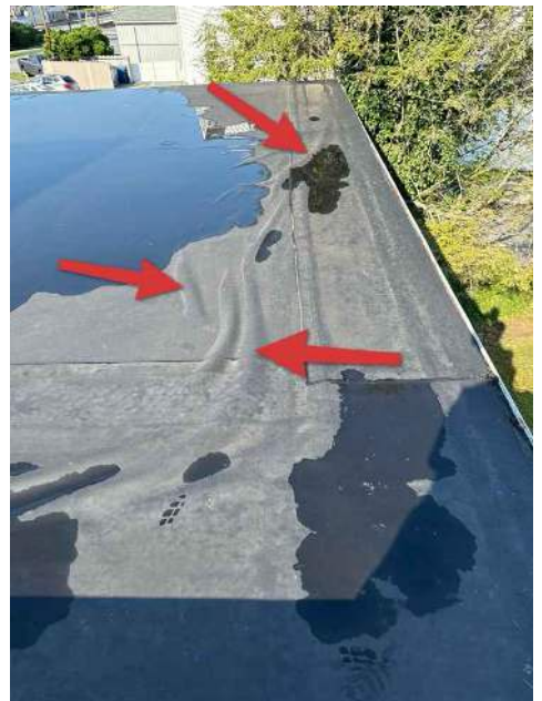
Visible wrinkles - sign that rubber has pulled back
