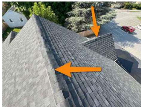
Architectural shingles used on ridge
