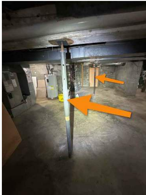
Split jacks supporting beams
