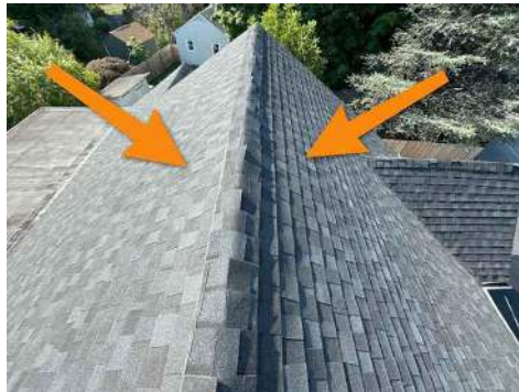
New roof installed over top of old roof
