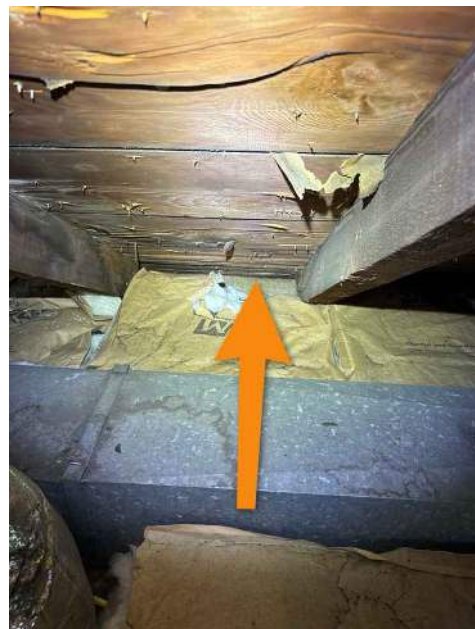
Does not appear to be any soffit vent
