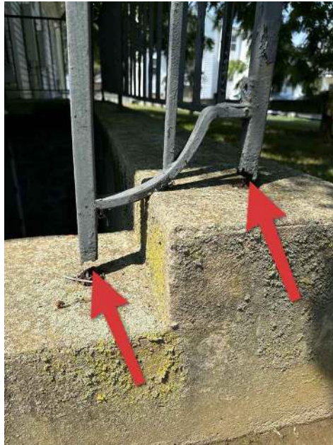
Rusted all the way through
