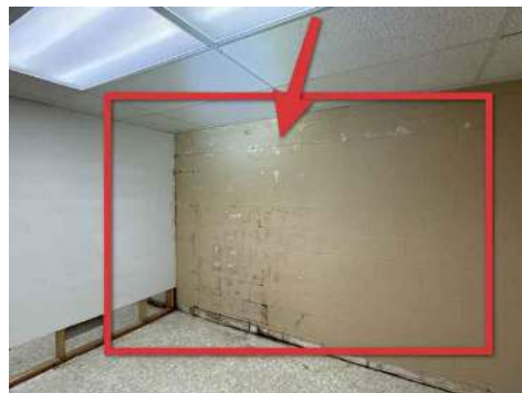
Moisture stains on rear basement wall
