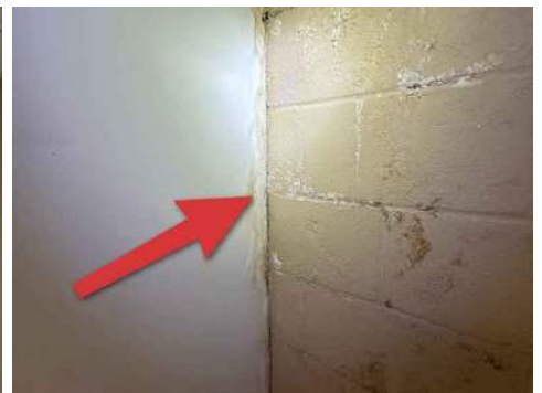
Close up of moisture stains on block and drywall
