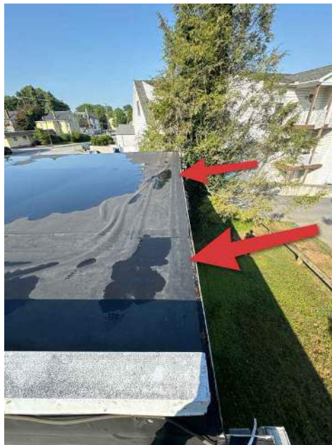
Edge of rubber, not sealed to roof
