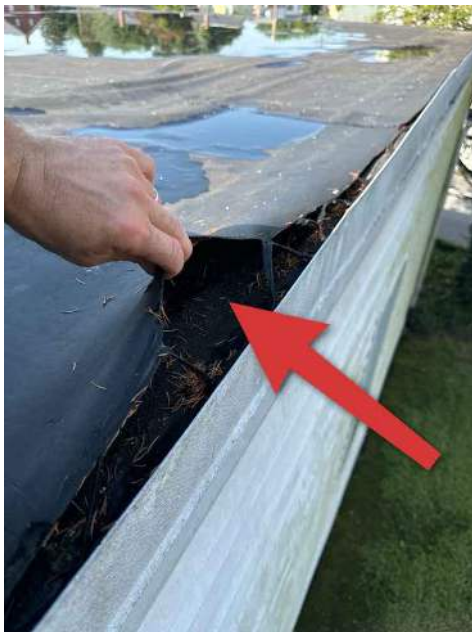
No adhesive at edge seam
