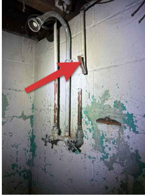
Waterlines cut and crimped
