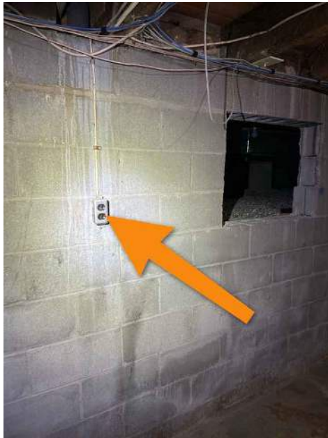
Upgrade from 2-prong to 3-prong receptacle
