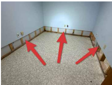
Base of finished walls removed
