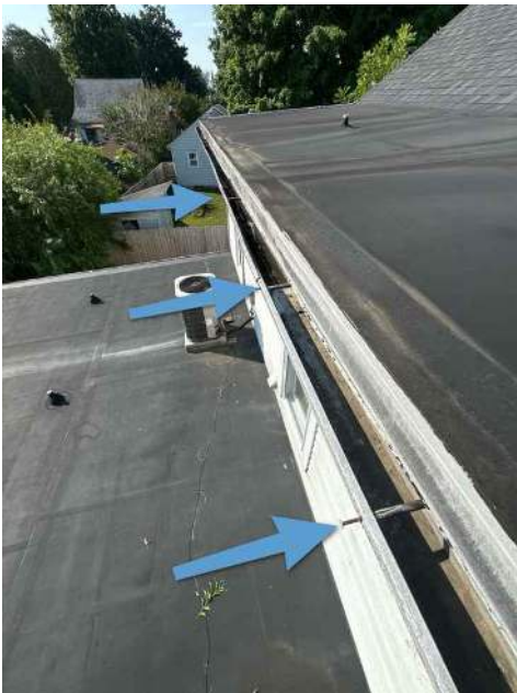
Gutter nails backing out
