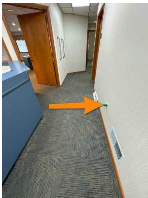
Reversed Polarity
