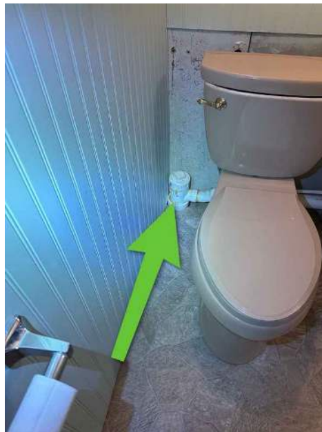
Rear Right Side Basement
