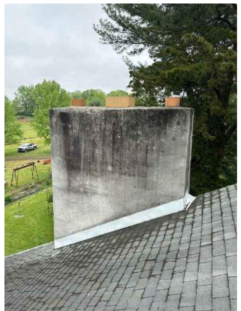
Right Side Chimney
