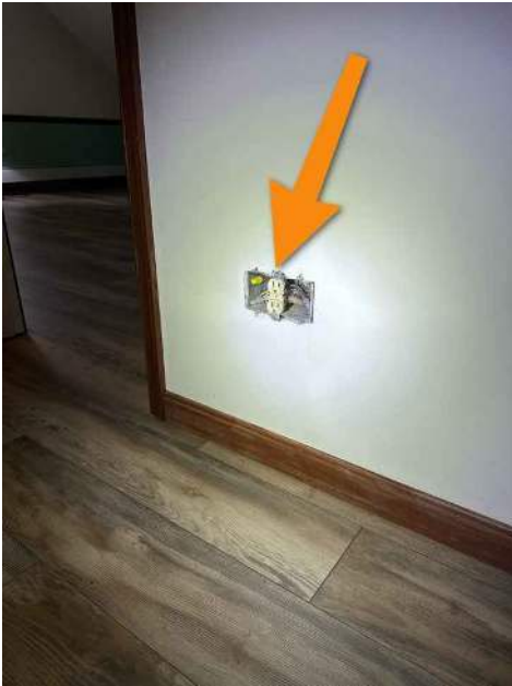
2nd Floor Hall
