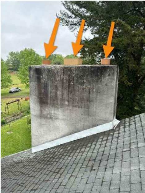
Right Side Chimney
