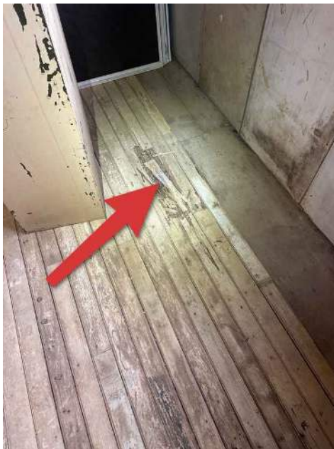
Floorboards deteriorated
