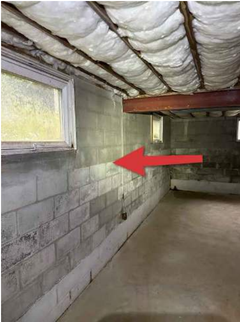
Left Side Foundation Wall
