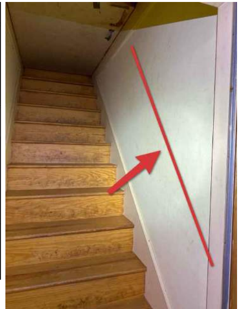
Stairs to attic
