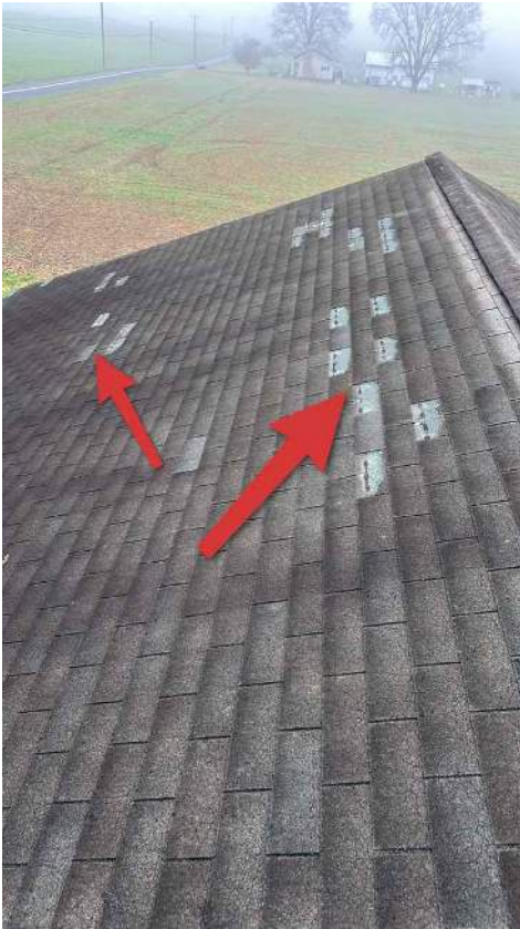
Missing shingles
