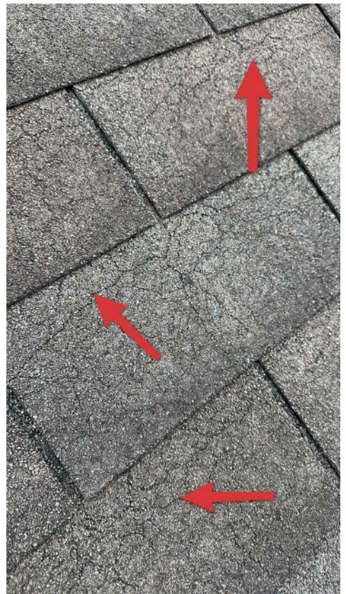
Extensive cracking
