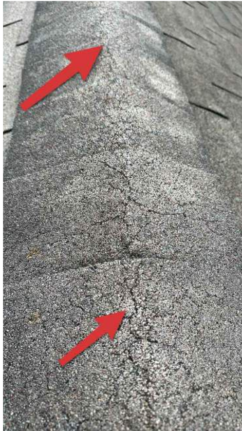
Ridge cracking
