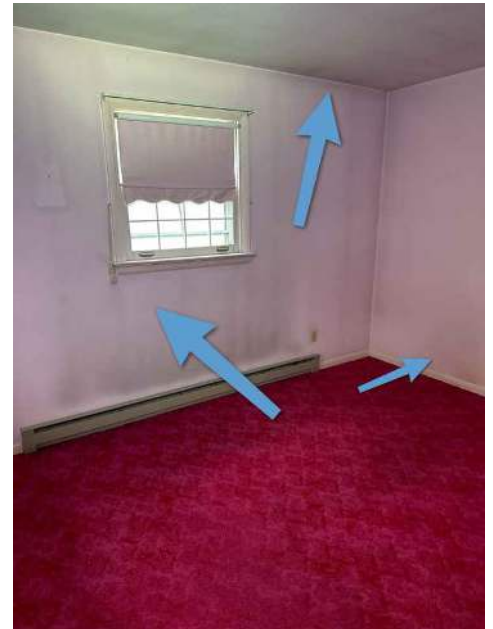
Representative of walls and ceilings
