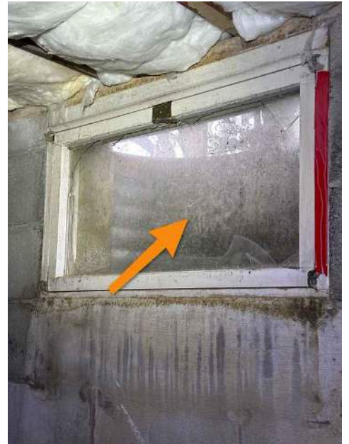
Front Basement Window
