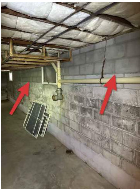
Rear Foundation Wall
