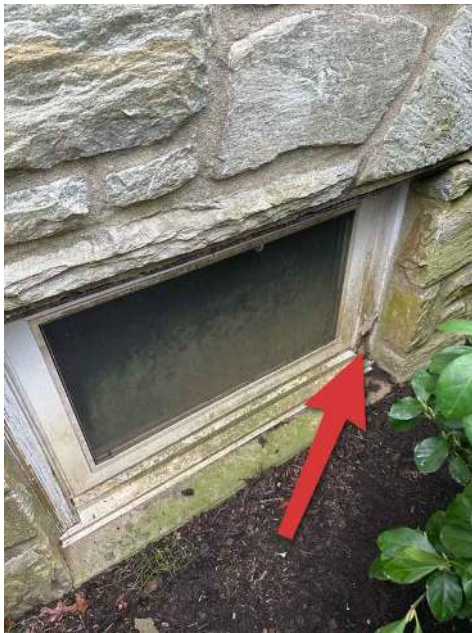
Left Side Basement Window trim
