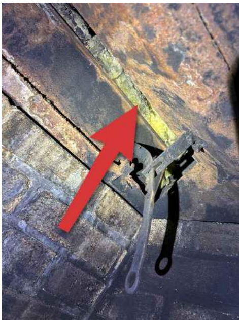
Insulation in flue Living Room
