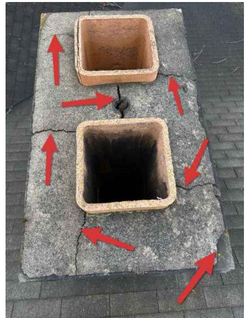
Extensive cracking
