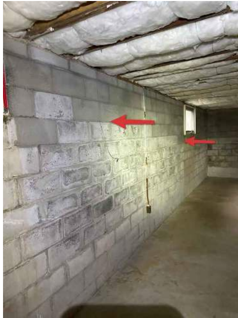
Front Foundation Wall
