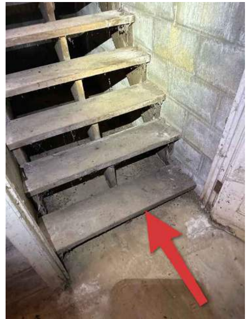
Basement access steps
