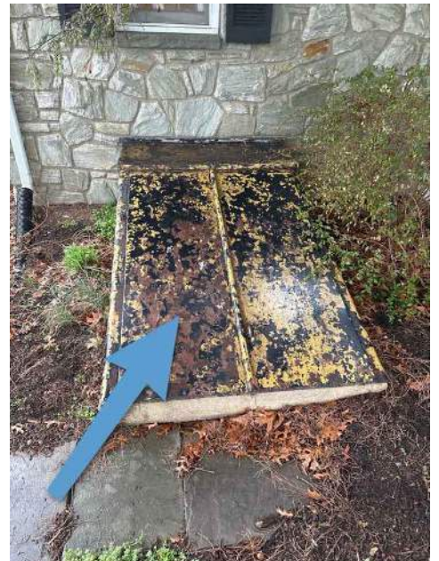
Rear Basement access
