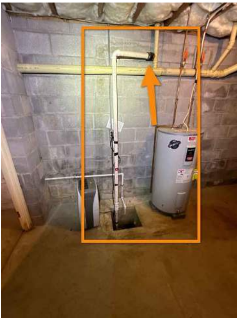
Drain to septic system
