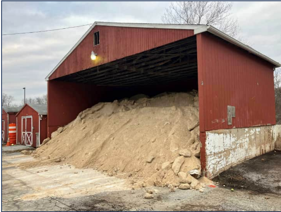
Salt storage shed
