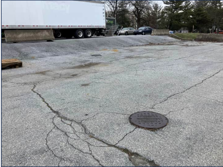
Sewer manhole on eastern portion of Subject Property
