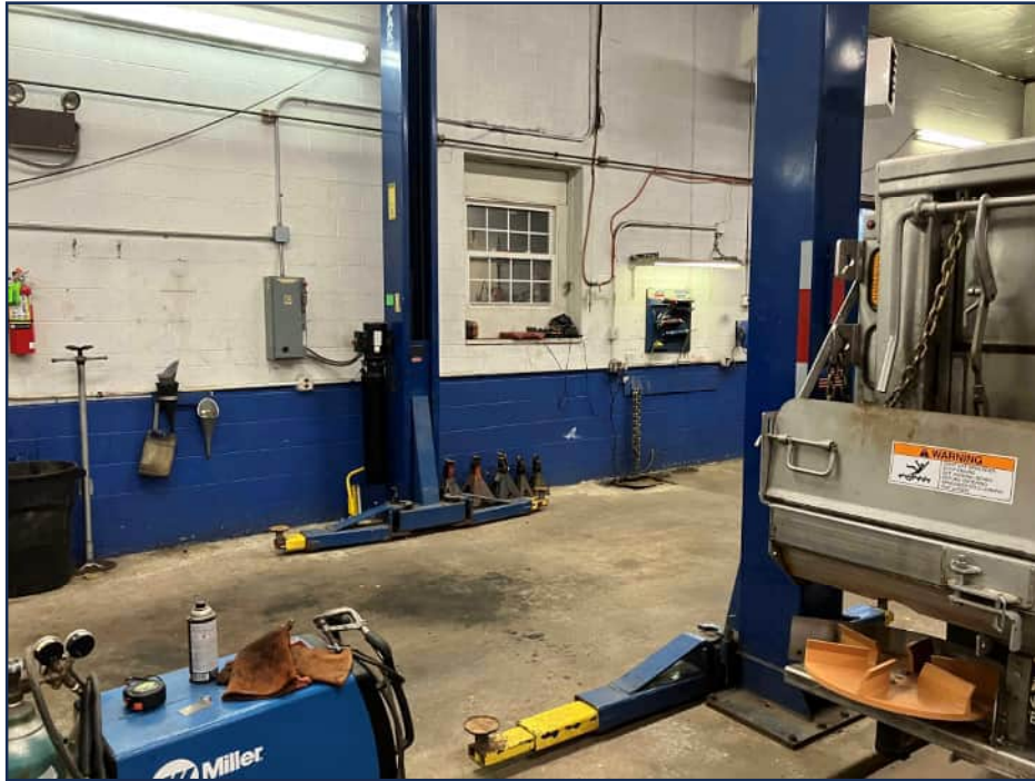
Shop area and above ground hydraulic lift in maintenance building
