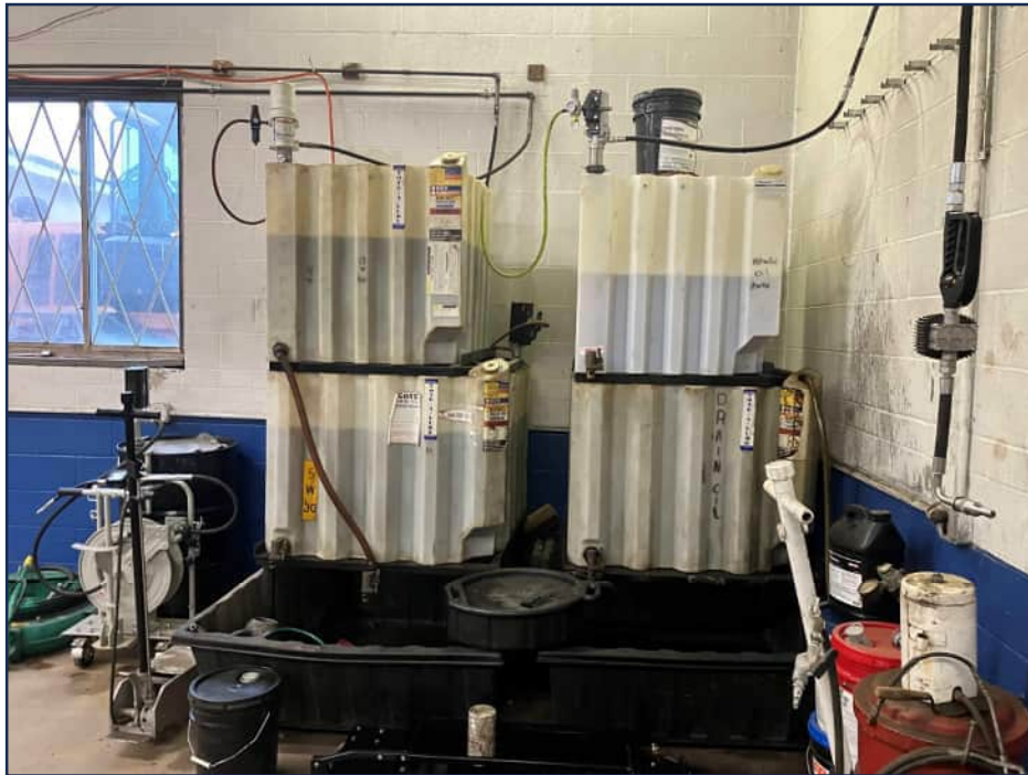
110-gallon hydraulic oil AST, 110-gallon motor oil AST, 180-gallon motor oil AST, and 180-gallon used oil AST in maintenance building
