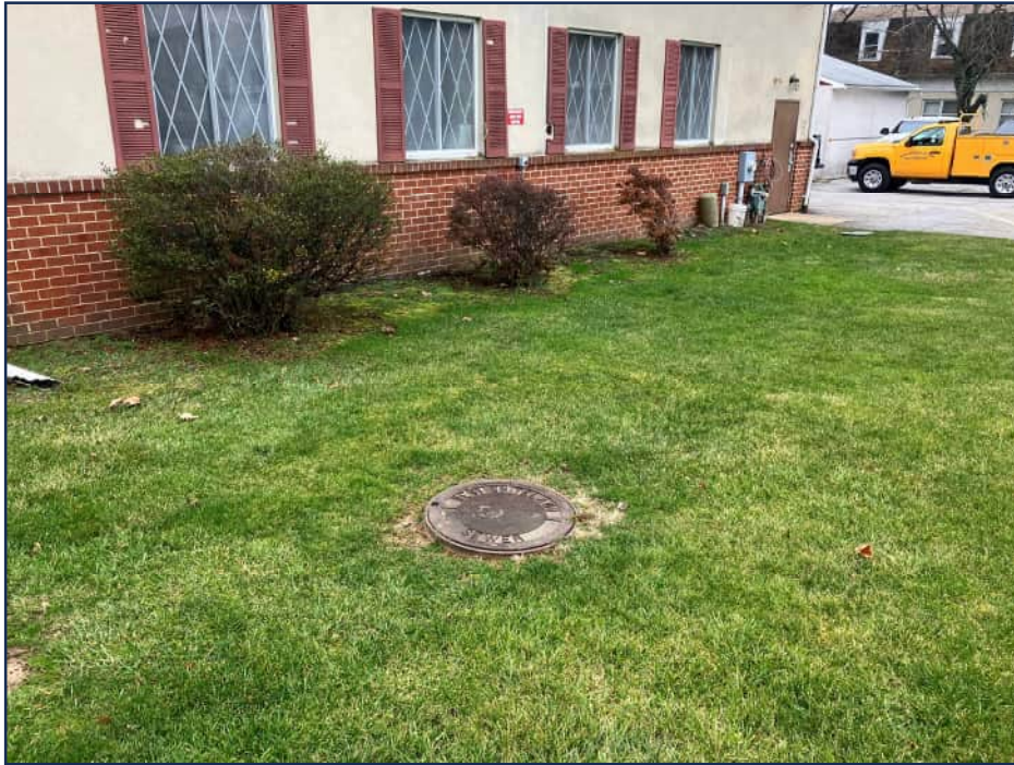
Septic tank manhole. Reportedly connected to leach field.
