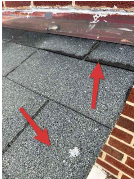
Close up of shingle wear
