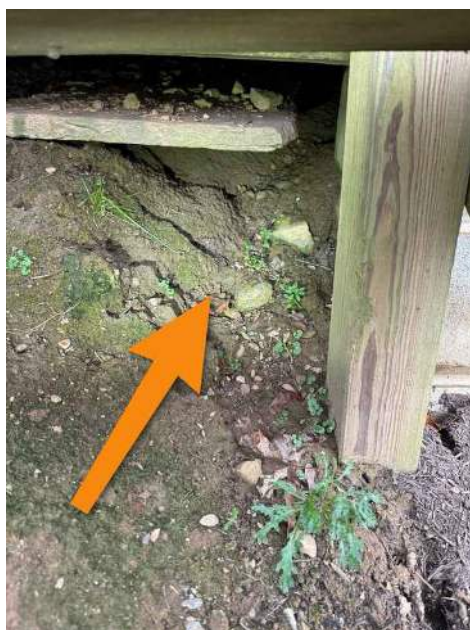
Erosion of soil under deck
