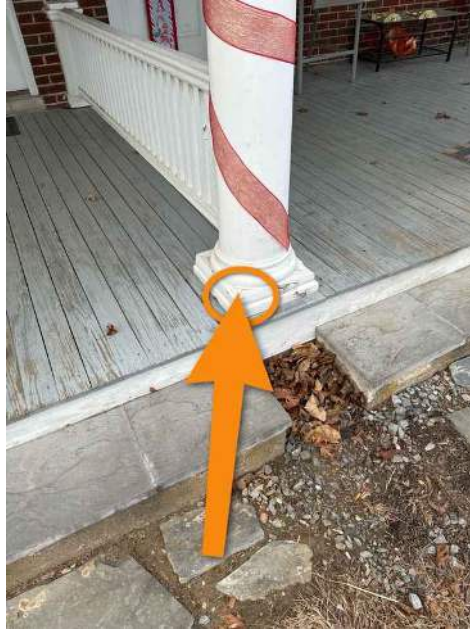
Rot beginning to develop at base of post
