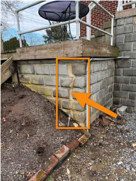
Past repair made to wall that pushed out
