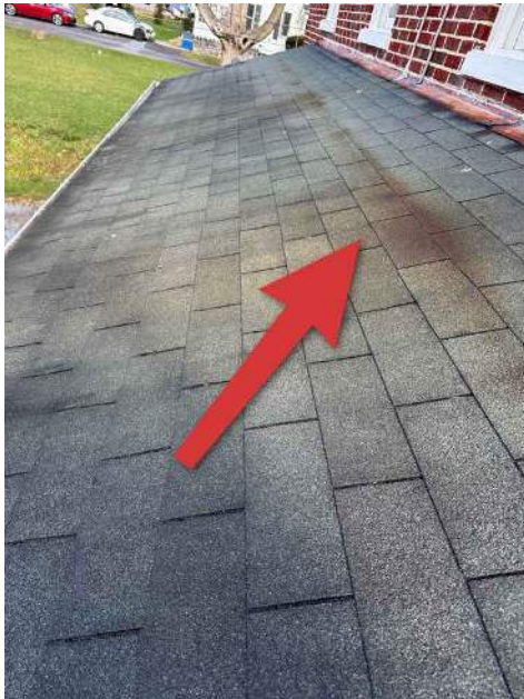
Rear Porch Roof shingles wearing thin
