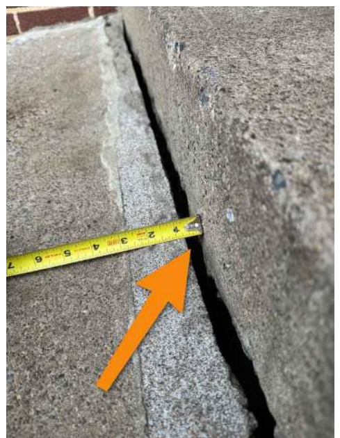
Gap separation at top of steps
