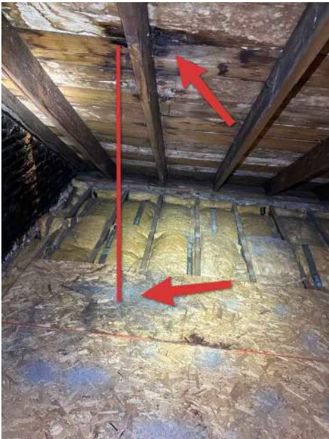
Leak at sheathing/deposit on floor
