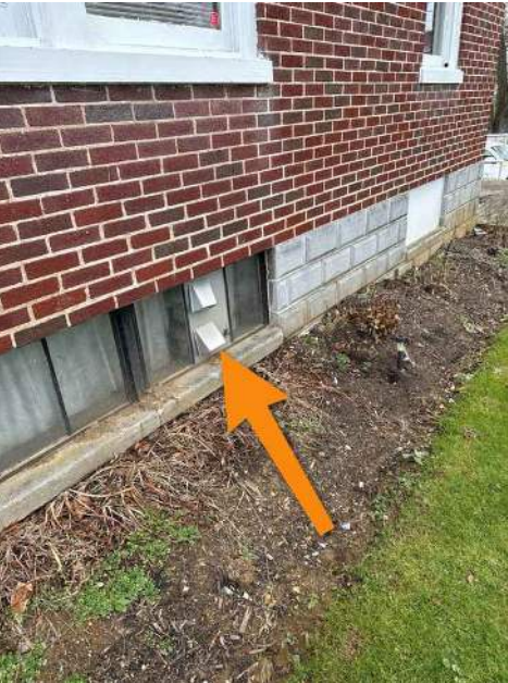
2088 dryer vent needs cleaned out
